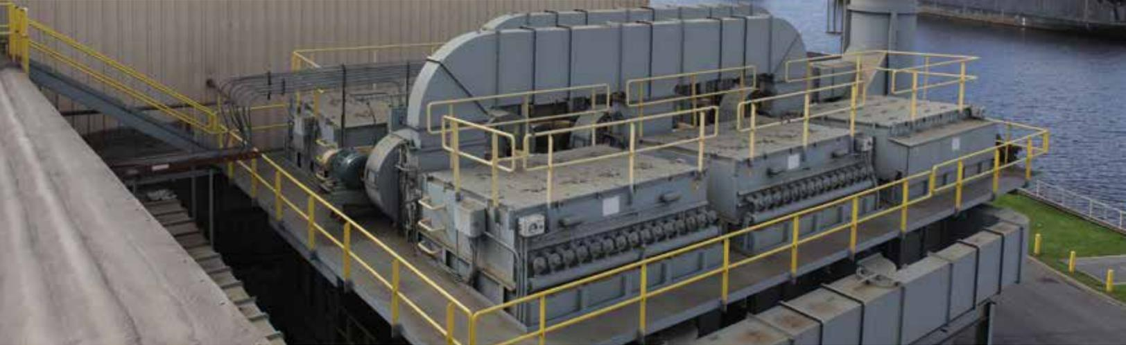
Creating thousands of castings per day can be a dirty job. Dust, sand and other particles move throughout the foundry air, but thanks to Waupaca Foundry's air-filtration system and advanced baghouse technology, we keep the air as clean as possible inside the plant and outside in the blue sky above.
