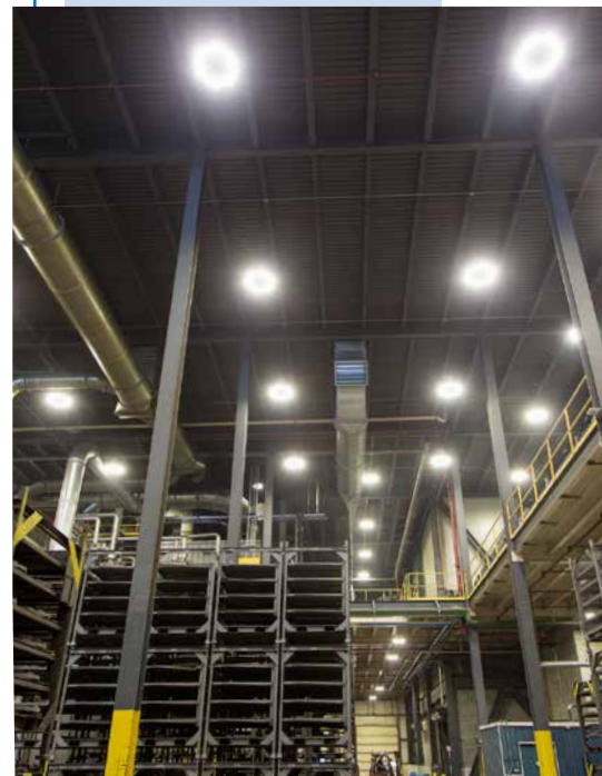
The core room expansion at Plant 1 utilized energy-saving LED fixtures throughout the production floor.
